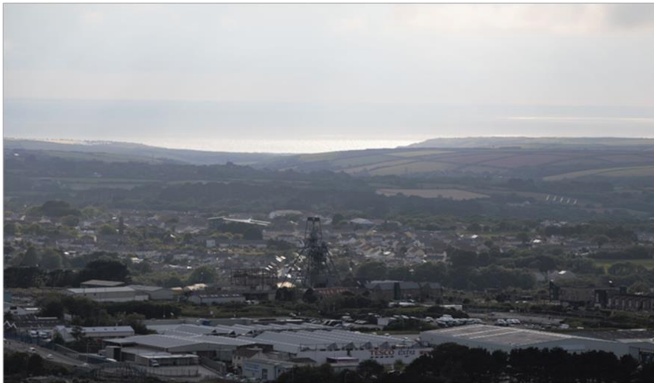
Figure 5.3 Photograph of the New Cook’s Kitchen headframe
