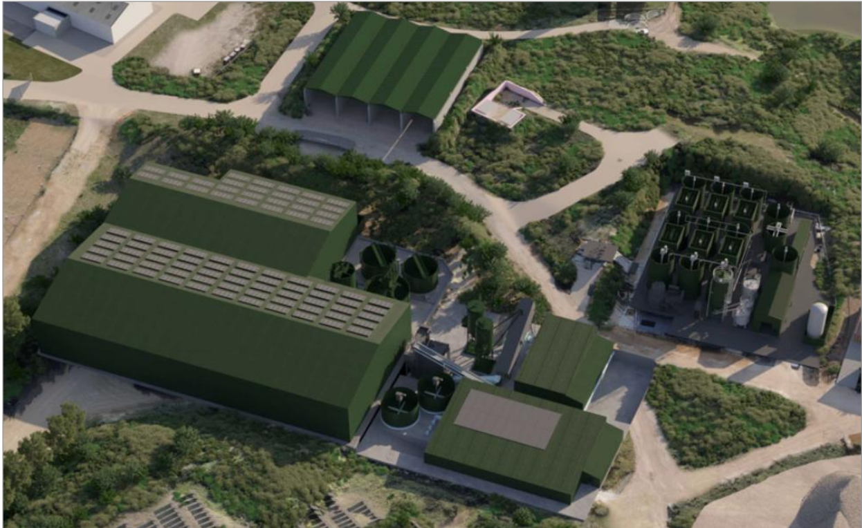
Figure 16.16 Backfill plant location (rendered image)
