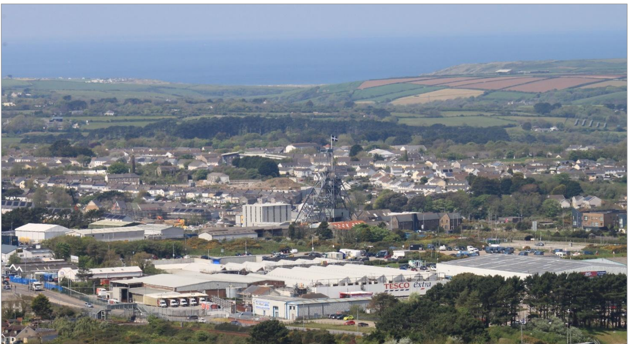
Figure 5.3 Photograph of the NCK headframe
